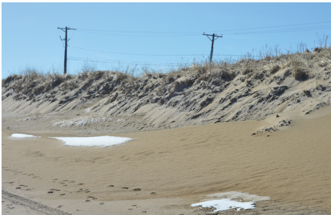
Figure 3.1 Sand dune erosion along Salisbury Beach
