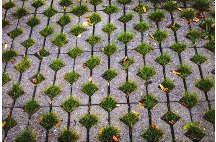
Permeable pavement provides gaps in impervious surfaces to increase stormwater absorption.
