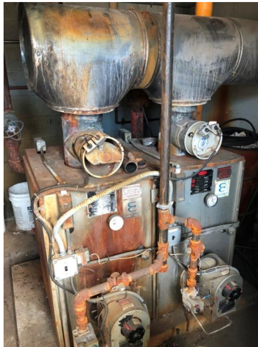
Figure 2: Existing Hot Water Boilers
