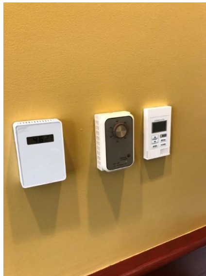
Figure 5: Controls Systems Present In Space; From Left to Right, CO2 Sensor for ERV, Thermostat for Boiler, Thermostat for Heat Pump.
