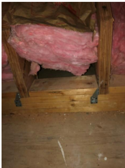
Figure 9: Insulation/Air Barrier Not Installed Continuously to Floor
