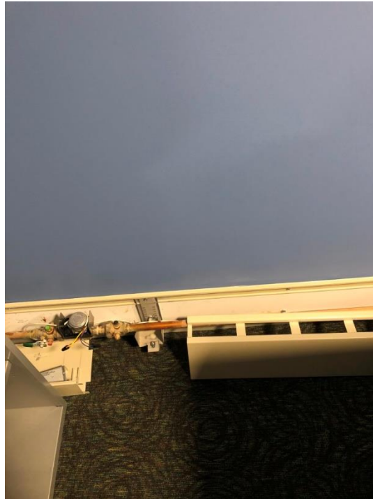
Figure 7: Missing Fins on Baseboard Radiator
