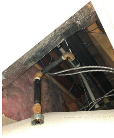
Figure 8: Sprinkler Piping Located in Space Open to Soffit Venting
