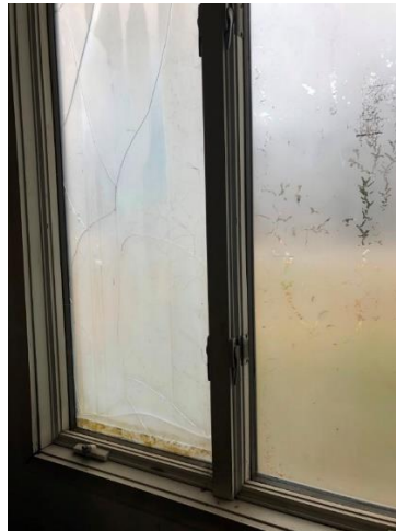
Figure 3: Window with Broken Seal
