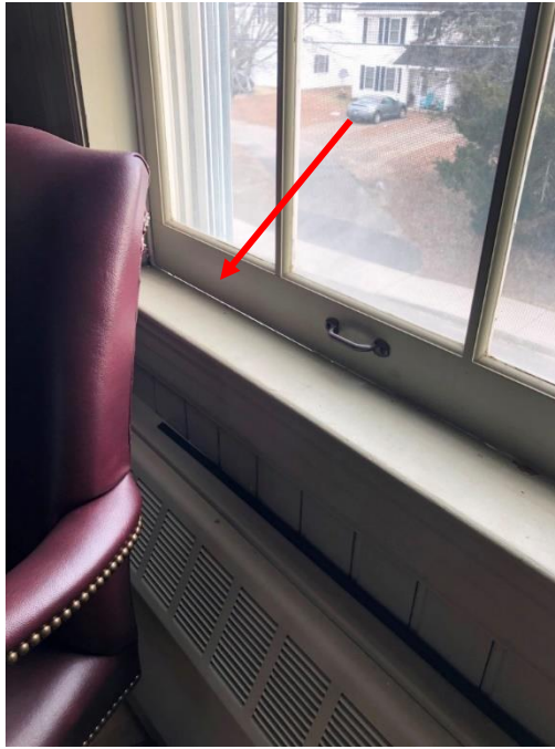
Figure 1: Air Gap in Second Floor Window
